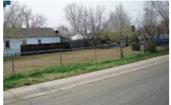
The sidewalk network in Westwood is inconsistent in quality and often too narrow for even two pedestrians to walk abreast.
