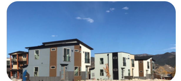
Chaffee Housing Trust uses factory-built modular homes to reduce the cost of homeownership in the rural resort communities near Chaffee County. Learn more at chaffeehousing.org .
